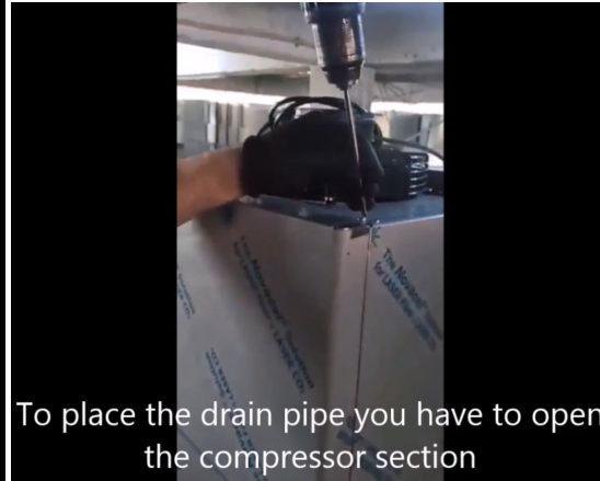
To place the drain pipe you have to open the compressor section
