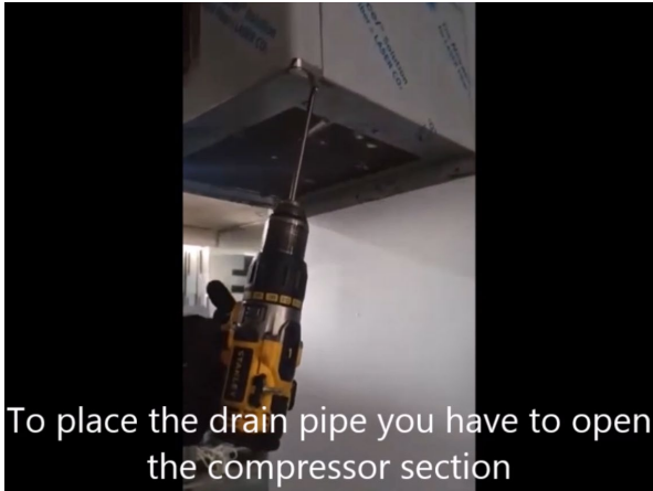
To place the drain pipe you have to open the compressor section
